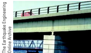
Bridge with roller support (see 1.1, 1.2)
